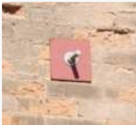
A steel plate with anchor bolts.
